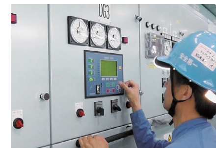
Inspection of high voltage switchboard
