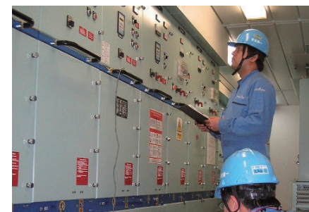
Inspection of motor protection relay
