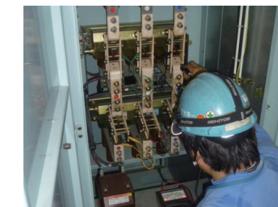
Insulation resistance check
