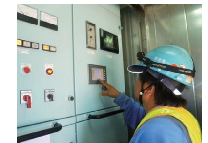
Alarm and status check
